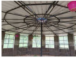
Canopy Roofing Structural Shade
