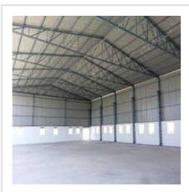
Structured Roofing Shade
