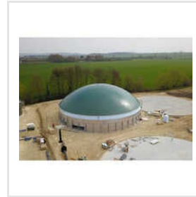
Biogas Power Generation Plant
