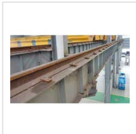
50 HRC EOT Crane Rail
