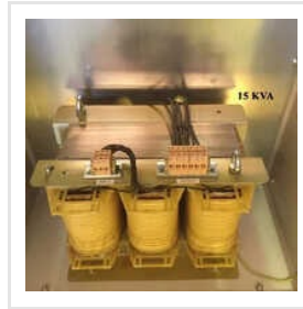
15 KVA Three Phase Isolation Transformer
