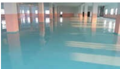
Pu Concrete Flooring Service
