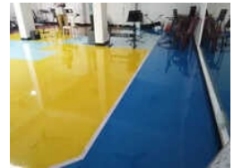
Epoxy Floor Coving Service
