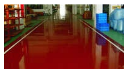
PU Self Level Flooring Service
