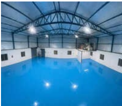
Industrial Epoxy Flooring
