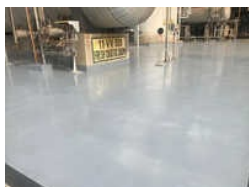
Epoxy Resin Coating Service
