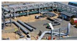
Mild Steel Pipeline Fabrication Services
