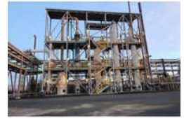
Structural Steel Erection Services
