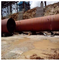
Pipeline Erection Services
