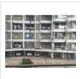
Pigeon Safety Netting Service
