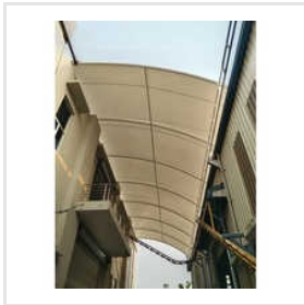
Top Area Tensile Covering Structure
