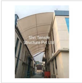
Tensile Walkway Structure
