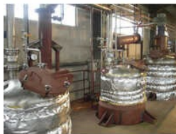
Semi Automatic Solvent Extraction
