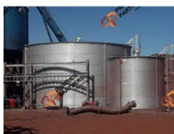
Zincalume Steel Overhead Water Tank
