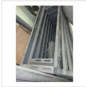
Elevator Combination Bracket
