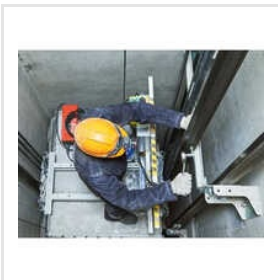
Passenger Elevator Installation Service
