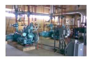
We offer wide range of Modular Refrigeration Packaged System Using different types of Compressors I reciprocating, hermetic, sealed, Scroll compressors with different types of gases as per requirement R22,R404a,R407C,R134a,R507A,R717(NH3)
