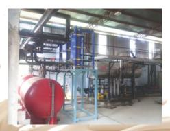
We design & manufacture L.P. Vessel packages, being used in refrigeration industries , as per customer's requirement. We do these packages on complete turnkey basis using all accessories like ammonia pumps, level controllers, 'Q'max & 'Q'min flanges, sight glass, valves, safety relief valve, strainers, oil pot etc.
