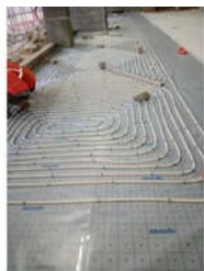
Radiant Underfloor Cooling System
