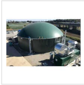
Bio Gas Dome Structure
