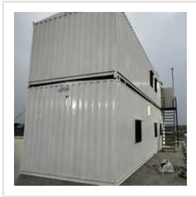
Steel Structure Site Office
