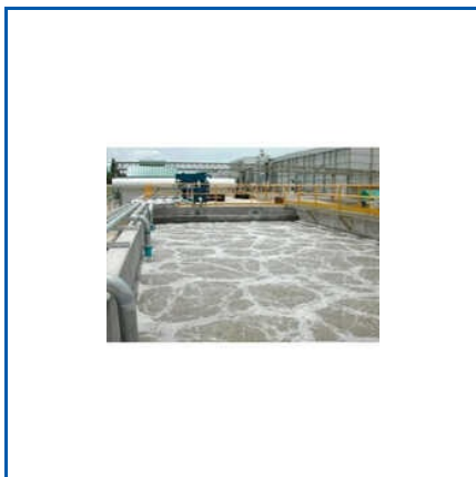
SLUDGE TREATMENT PLANT
