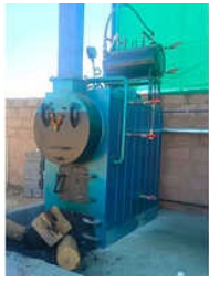
Non IBR Steam Boiler
