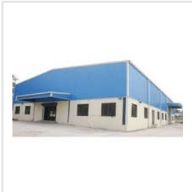
Industrial Mild Steel Shed
