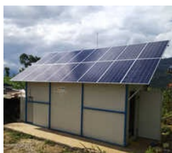
Solar Cold Storage
