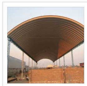
Mill Trussless Roof
