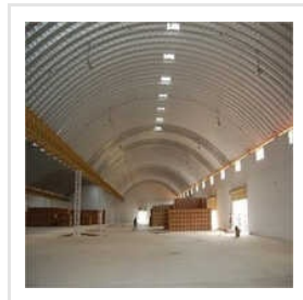
Metal Roofing System
