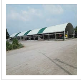
Truss Less Roofing Structure
