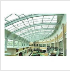
PEB Structural Steel Shed
