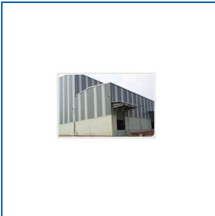
PEB STEEL STRUCTURE CONSTRUCTION SERVICE
