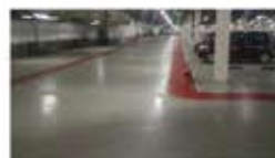
Epoxy Flooring System For Car Parking
