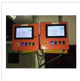
Robotic Chassis Visual Inspection
