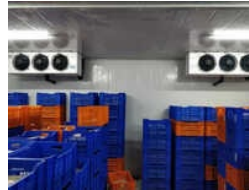
Cold Storage Room
