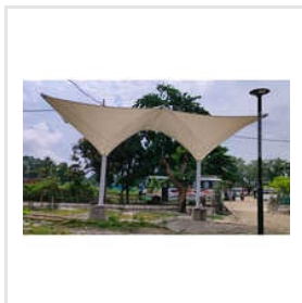
Inverted Umbrella Tensile Structure
