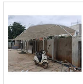
PVC Curve Tensile Shed Structure
