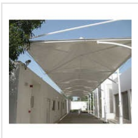
Industrial Tensile Structure
