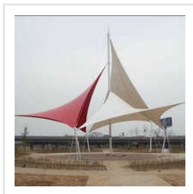
Skyler Tensile Structures
