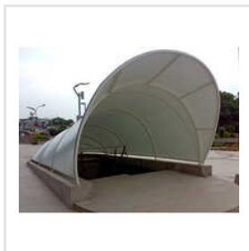
Tensile Walkway Structure
