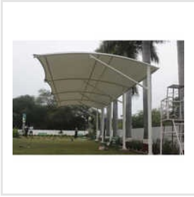
Tensile Fabric Structures Shed
