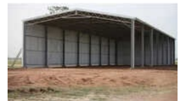
Mild Steel Prefabricated Factory
