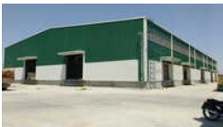
Pre Engineered Building Structure
