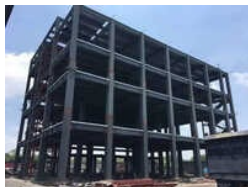
Pre Commercial Building Structure
