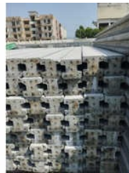
Precast Compound Wall Pillar
