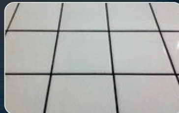
GROUTING WITH EPOXY & CEMENTIOUS GROUT
