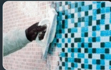
GLASS MOSAIC FITTINGS&GROUTING
