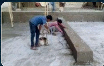
INJECTION GROUTING (CEMENTIOUS ,EPOXY&PU)
