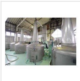
Vacuum Distillation Plant
