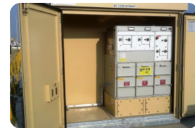
PSS WITH MV SWITCHGEAR/RMU
