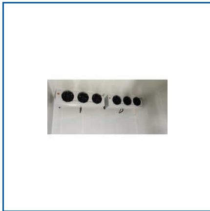
INDUSTRIAL BLAST FREEZER
