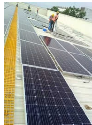
Industrial Solar Power Systems Installation
