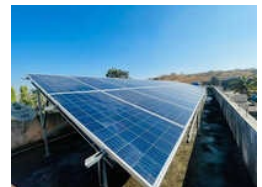
Solar Power Installation Services
