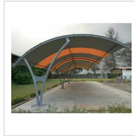
Car Parking Tensile Structure
