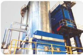
Hot Water Generator Solid fuel fired - up to 15 M Kcal/hr
