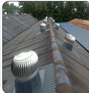
ROOF VENTILATORS WITH FRP GELCOTAE BASE
