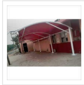
Car Parking Sheds
