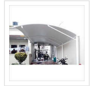
Car Parking Sheds
