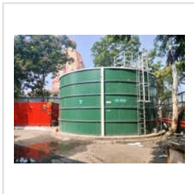
Industrial Fire Steel Tank
