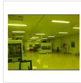
Clean Room Construction Service
