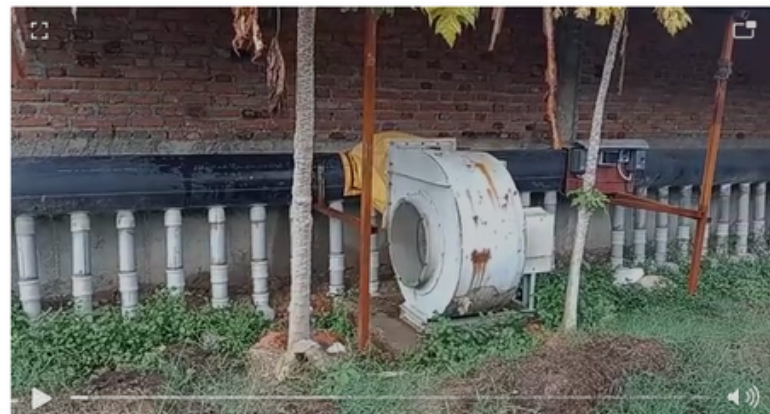
Machines and materials used
