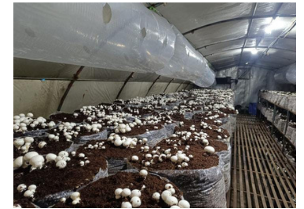
Polythene Air Distribution Ducts
