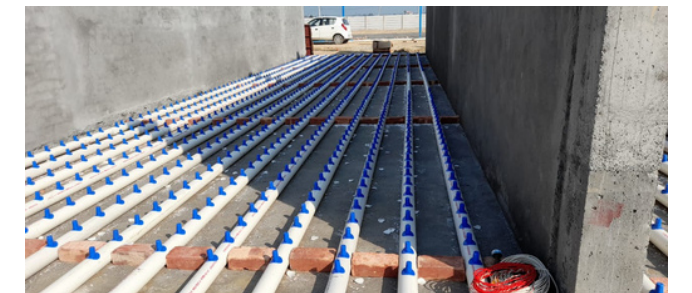
Spigots (air diffusers)
