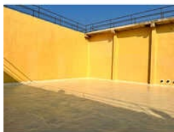
Epoxy Tank Coating Service
