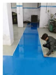
3 MM Epoxy Flooring Service
