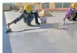
Roof Coatings Service
