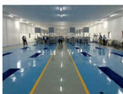
1 MM Epoxy Flooring Service
