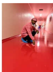
Epoxy Flooring Service
