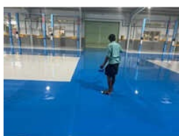
2 MM Epoxy Flooring Service
