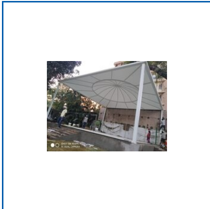
MARRIAGE HALL TENSILE STRUCTURES
