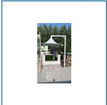
FABRIC GAZEBO TENSILE STRUCTURES
