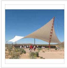
Fabric Tensile Membrane Structure
