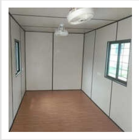
Internal Container Cabin
