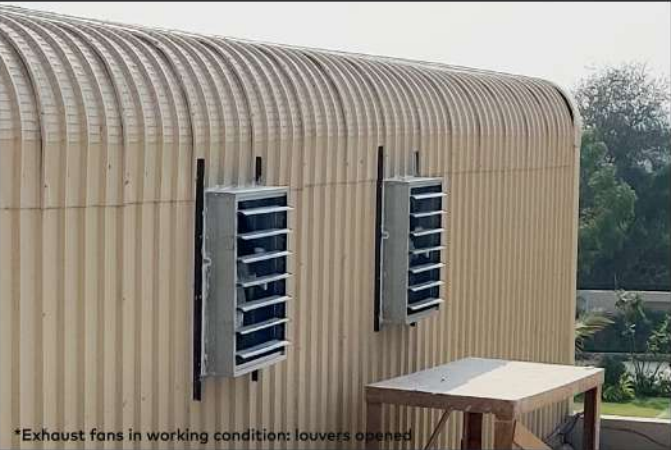
*Exhaust fans in working condition: louvers opened
