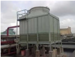
2400 X 2400 X 3200mm Frp Cooling Towers
