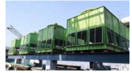
200TR Frp Industrial Cooling Tower
