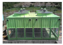
Waste Heat Removal Cooling Towers
