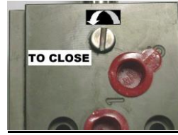
Manual Override "ON" Photo – 3
