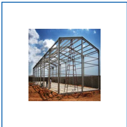
FACTORY SHEDS FABRICATION SERVICES
