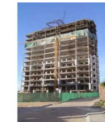
Industrial Building Construction Service
