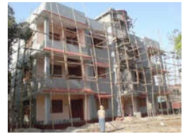
RCC Structure Service
