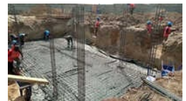
Foundation Construction Service
