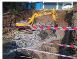
Mass Excavation Construction Service
