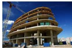
Industrial Building Construction Service
