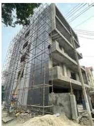
Hotel Building Construction Service
