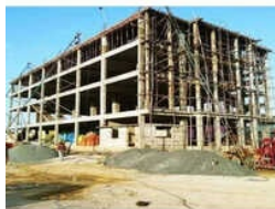
School Building Construction Service
