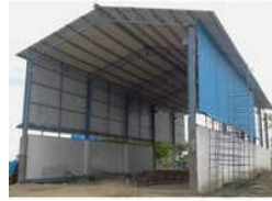
Industrial Prefabricated Factory
