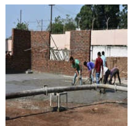
Commercial Building Construction Services
