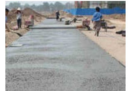
Concrete Road Construction Service
