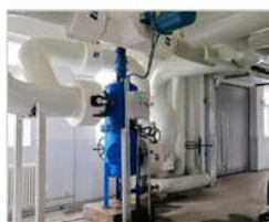
Self Cleaning Filtration Plant
