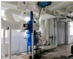
Self Cleaning Filtration Plant
