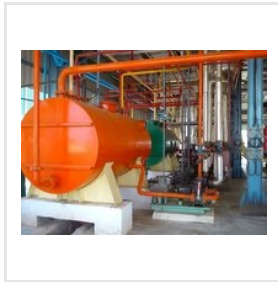
Solvent Extraction Plant
